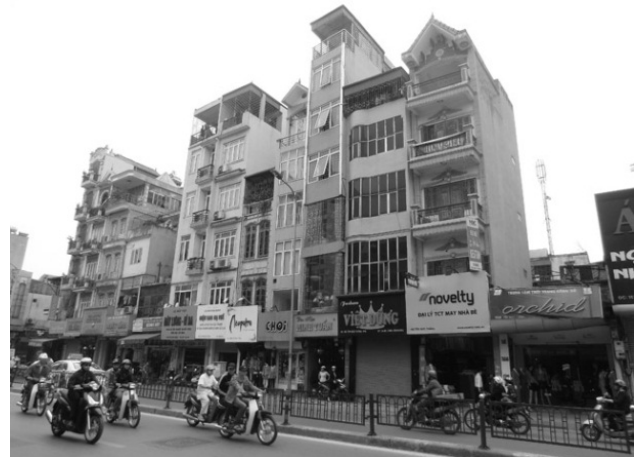
Fig. 5. An image of shop-house style buildings in Hanoi.
